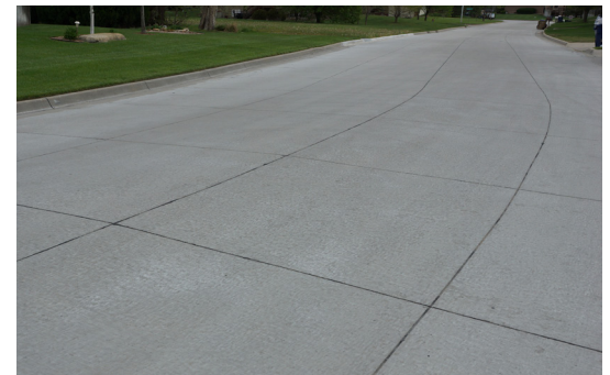
RCC Sample Crack Control Pattern
