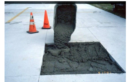
RCC Concrete Patch
